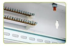
**TERMINAL BLOCK PE + N** Part of the cabinets are terminal block for connecting the PE and N wires and screw for main grounding point.
